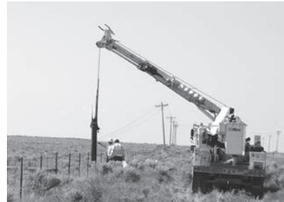
MCREA line crews replace a broken pole on Highway 71 south of Brush.
