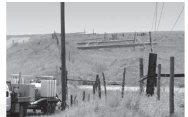
Linemen from the City of Fort Morgan work around debris and damaged structures to restore power along Morgan County Road Q south of Brush.
